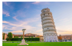
Leaning Tower of Pisa
